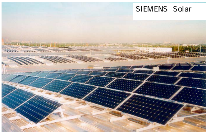
Fig. 7 Photovoltaic generator at the Munich Trade Fair 1 MWp, 1000 MWh/a, 7800 m 2 solar cells
