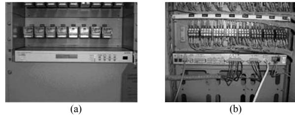
Fig. 2. Analyzer Power Sentinel 1133A installed in the substations Guamá and Utinga; (a) Front panel; (b) Back panel.
